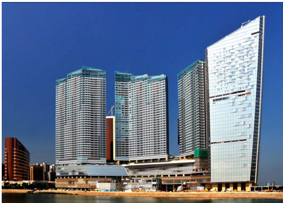
Fig 6: Construction of One Central is well advanced
